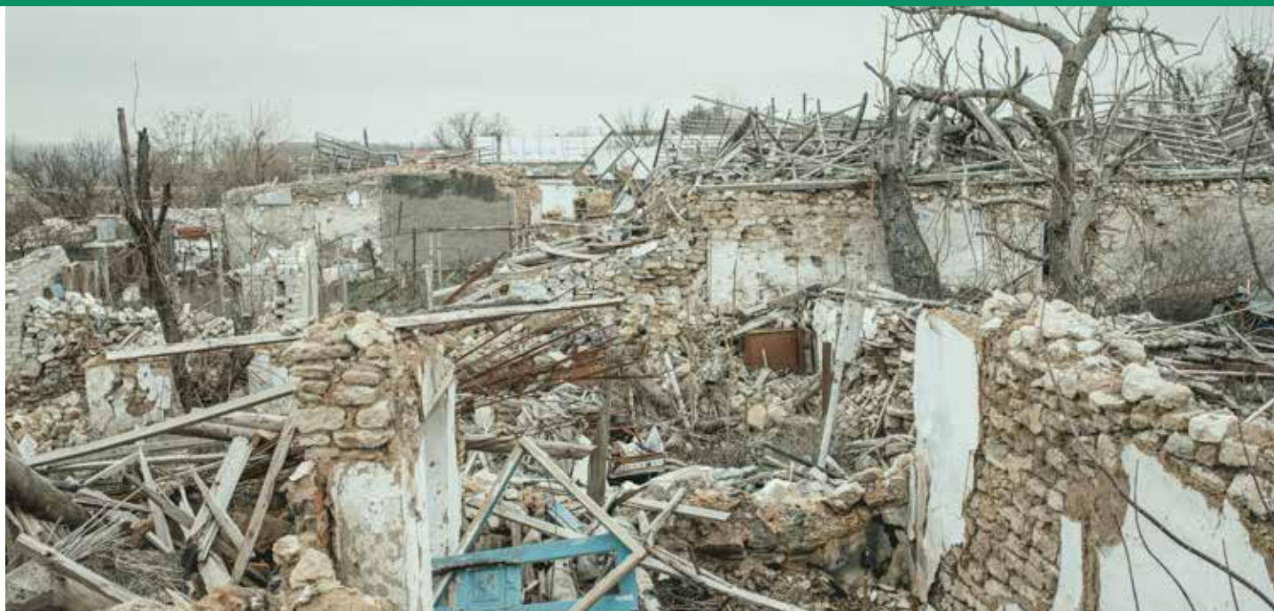
Destroyed residential buildings in Snihurivka, Ukraine. Credit: imageBROKER
