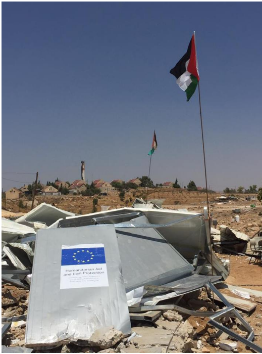
Demolished home in Umm al-Kher. Photo by Fadi Aroui. (See photo credits .)
